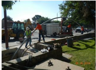
Carver Electric and their subcontractor bored and pulled in the IPP transformer conduit on Saturday 05/17. This conduit went under the Tunnel and two 24" chilled water conduits without a problem. This work is in preparation of going on-line with permanent electrical power to the Institute for Public Policy by 05/31. The conduit run is 180 feet long, depth is 15 feet with a 550 turn on the conduit going into the Astronomy electrical vault (shown in picture).
