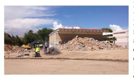
Demolition at Hardman Hall continues in order to make way for the Hardman and Jacobs Undergraduate Learning Center. The center portion of Hardman will remain to become updated active learning classrooms above and below. The steel is being separated from the concrete in order to recycle both materials, thus contributing to the sustainability efforts. The building is slated to receive a USGBC LEED Silver certification or above.
