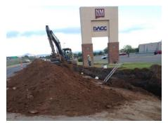
Also underway is the installation of a 24" diameter domestic water line on the east side of Sam Steele Way from Well 17 to Well 10 is scheduled to be completed in early September.
