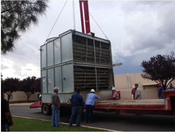
Tower replacement at DACC
