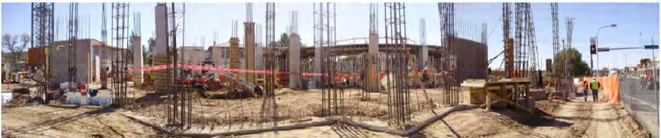
View from the Northeast corner of site
