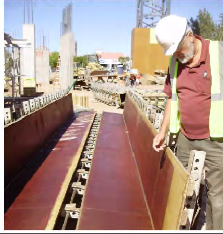
New square column form
