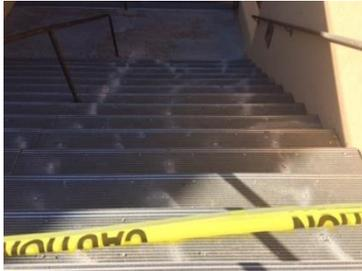
Structural Maintenance repaired the east exterior stairs of Corbett Center this week. They inspected all of the stair treads and secured the loose treads to the concrete stairs. Loose stair treads were a safety hazard and this repair provides a safe walking surface for the students and community members entering Corbett Center.
