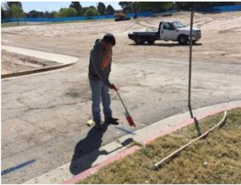
Utilities Shop personnel were locating the underground utilities, sewer, water, gas, power and lighting at the Monagle Hall demolition site. This work was part of the construction support to install a new irrigation system for landscaping the area. A contractor was tasked with excavating a six inch water line to cap. Capping the water line allowed the Shop to return service to a fire hydrant and an irrigation backflow that is required for the irrigation system.
