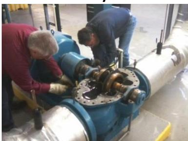
Central Utility Plant employees performed a scheduled preventive maintenance inspection on chilled water pump #3 in the Central Utility Plant. During the inspection, they identified a leaking seal that required replacement. They scheduled an overhaul of the pump which included replacement of the bearings and seals. Their efforts ensure that the pump is ready for service during the cooling season. This is one of several pumps providing cooling to
