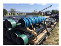
Facilities and Services Utilities Department is currently installing over 200 feet of new column pipe and pump bowl assemblies as part of an ongoing water well refurbishment project. Enhanced water level monitoring instrumentation will also be installed which will provide valuable information on any changes to the water table during well operation. Camera inspections of the well casing and filtration screens indicate that this well should provide many more years of
