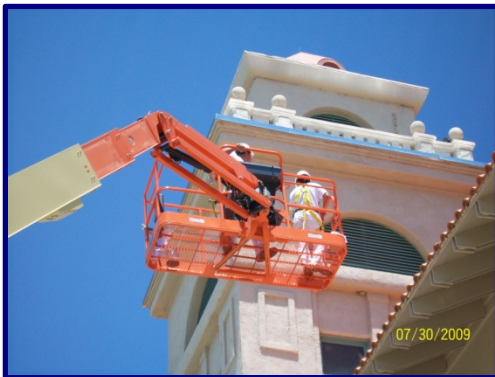
Goddard Tower emergency repairs
