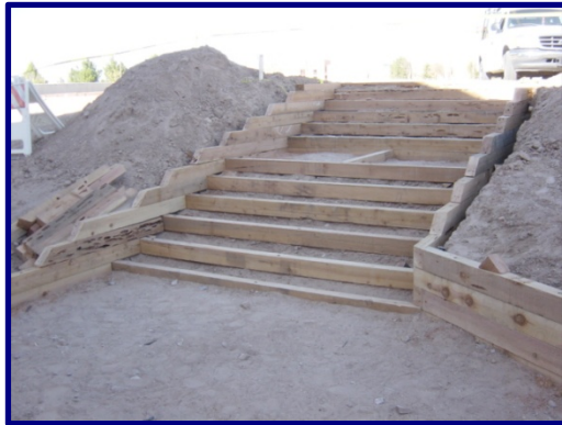
Walkway and stairs at Chamisa
