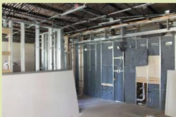
Blue jean insulation in all interior and exterior walls
